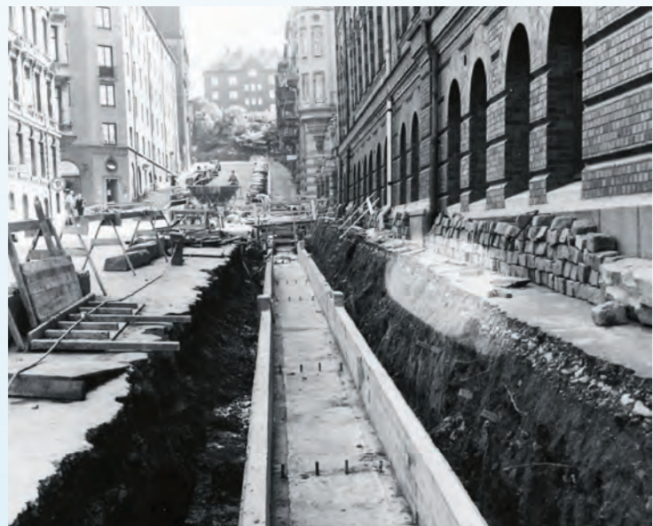
Finished concrete culvert
