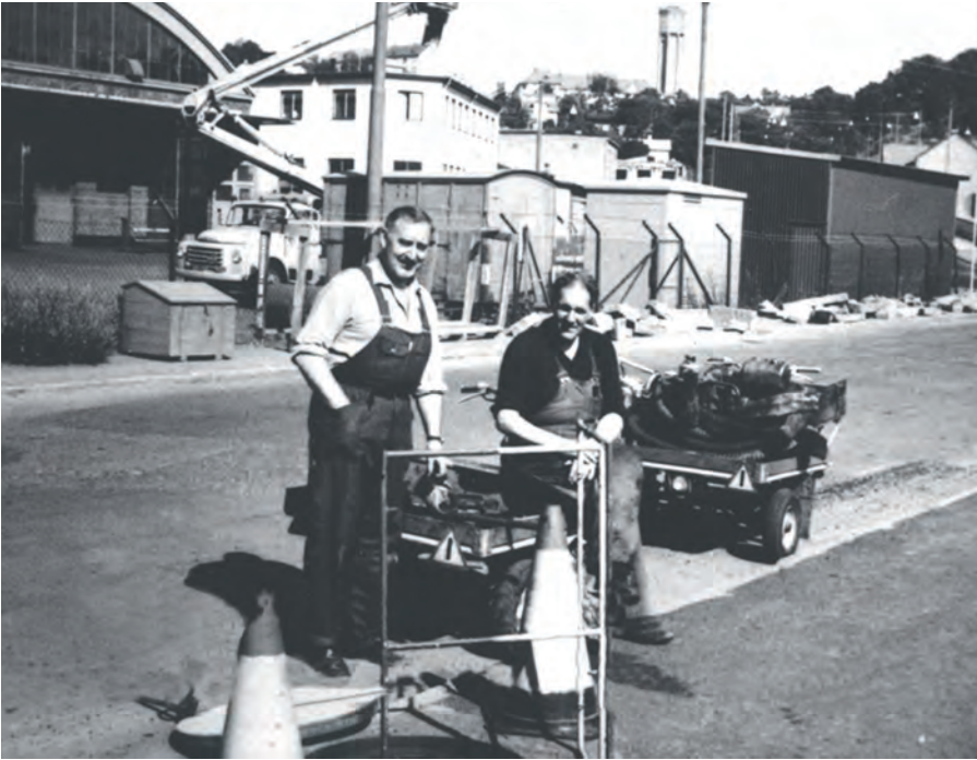
Maintenance tools for the district heating system were transported with mopeds in the 60's
