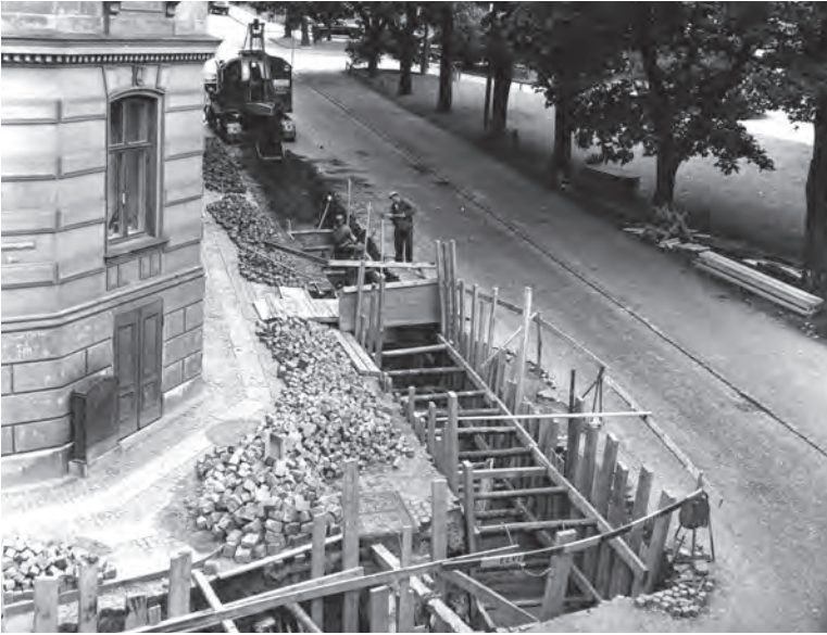
Network construction in the Haga Kyrkogata and Bellmansgatan intersection
