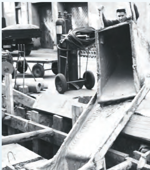
Casting culvert covers
