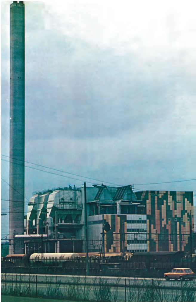
The waste incineration plant (1971)
