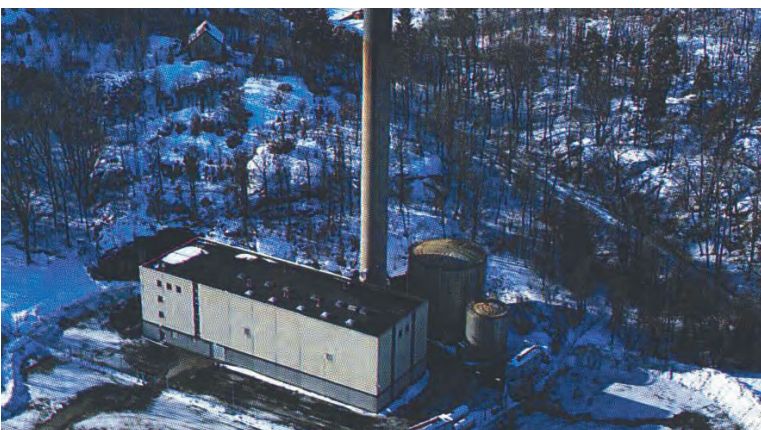
The plant in Angered – initially supplying a separate district heating network with heat
