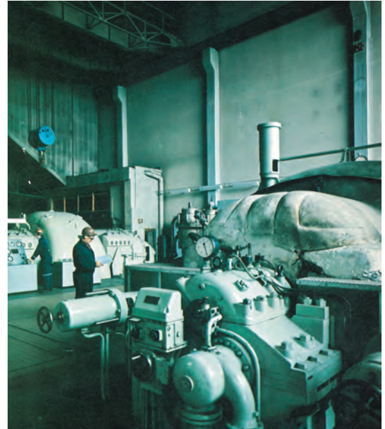
The turbines at Rosenlund, one of the Combined Heat and Power plants (1973)
