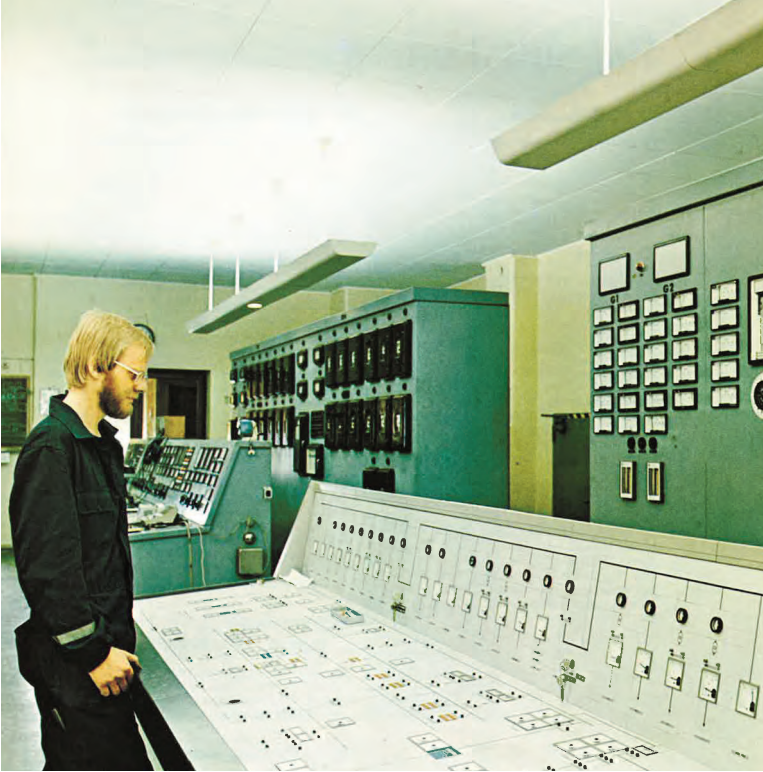
Rosenlund, control room (1974)
